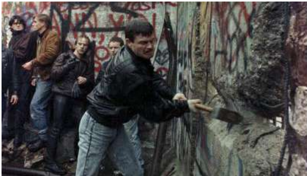
Demolition of Berlin wall
